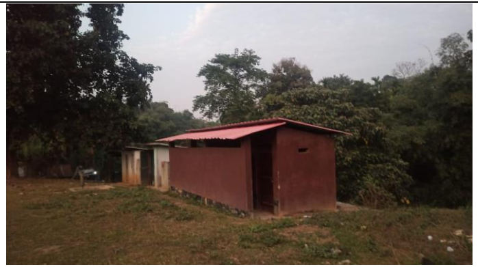
fig: Toilet facility in the market area
